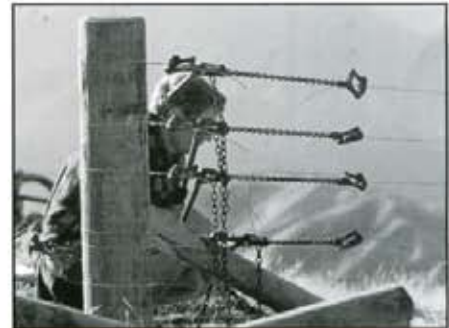
END STRAIN Tie off wire to strainer post using wire strops.
