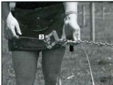
3: Take up the slack in the wire and attach remaining grip [3].
