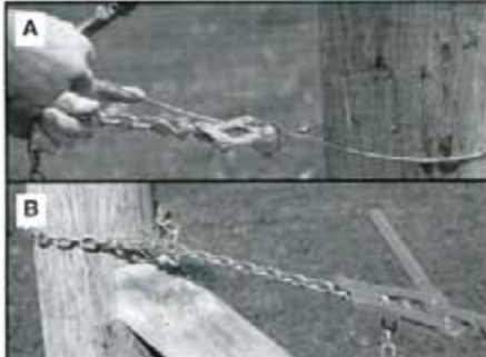
END STRAIN Place a wire strop (A), or anchor chain H113 (B), around strainer post. Attach chain to grab, remove slack in wire and place in grip.
