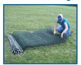
With the folds on the ground, roll the netting toward the posts and retie the bundle with the green strings.
