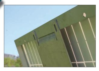
Once bracket is secured to the post, slide panel into the top of the bracket. This will safely hold the panel in place while self-tapping screws are attached.
