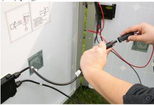
**Step 5:** Connect Panel B's negative (top) plug to the charge controller's negative (black) plug.
