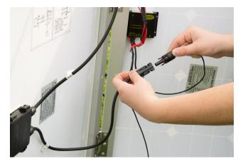
**<u>Step 4</u>:** Connect Panel A's positive (top) plug to the charge controller's positive (red) plug.
