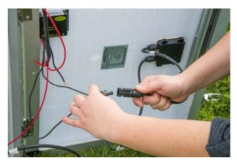
**<u>Step 6</u>**: Connect Panel B's positive (bottom) plug to the charge controller's positive (red) plug.
